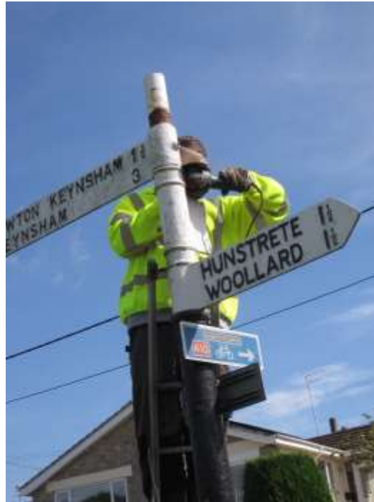
Starting to remove the 1 st finger
