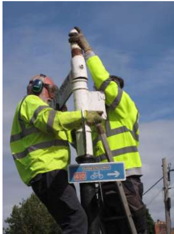
Removing the 1 st finger
