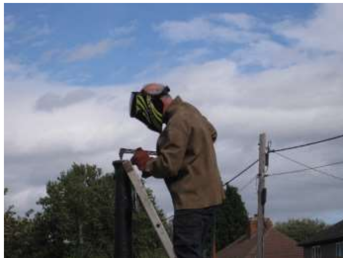
Gas cutting to remove the remains of the inner post
