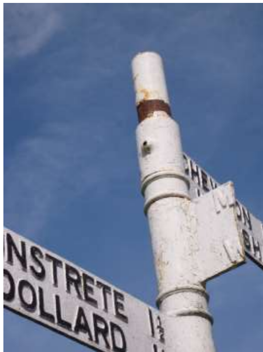
Finial has been removed
